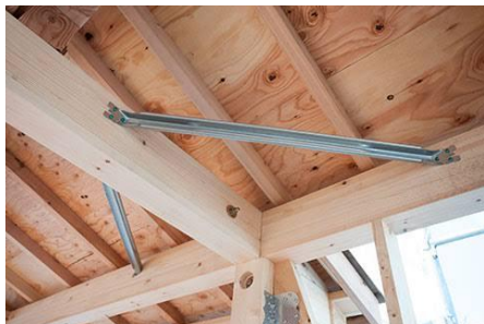
Seismic strengthening in a house.
